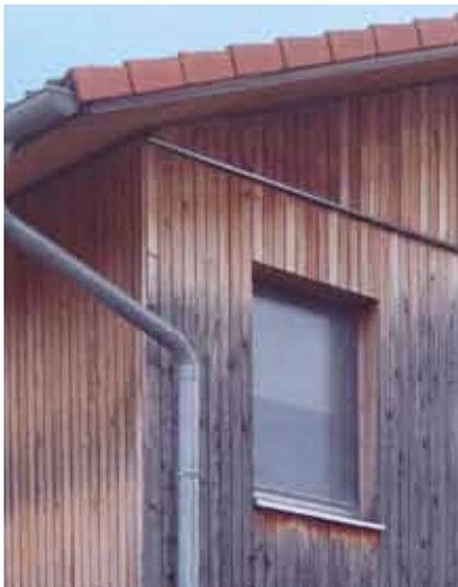
Untreated wooden facades change their colour and texture under environmental influences. It is difficult to predict such changes because many factors influence the different facade surfaces of the building exposed to the weather in various ways. Such as wood type, location, direction, air purity and
